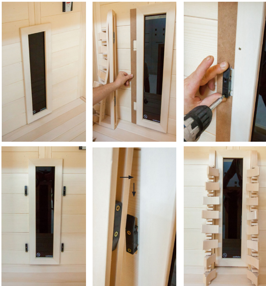
Fig. 29: Installing the backrests
