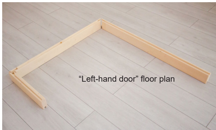
Fig. 1: Laying the three base frame elements
